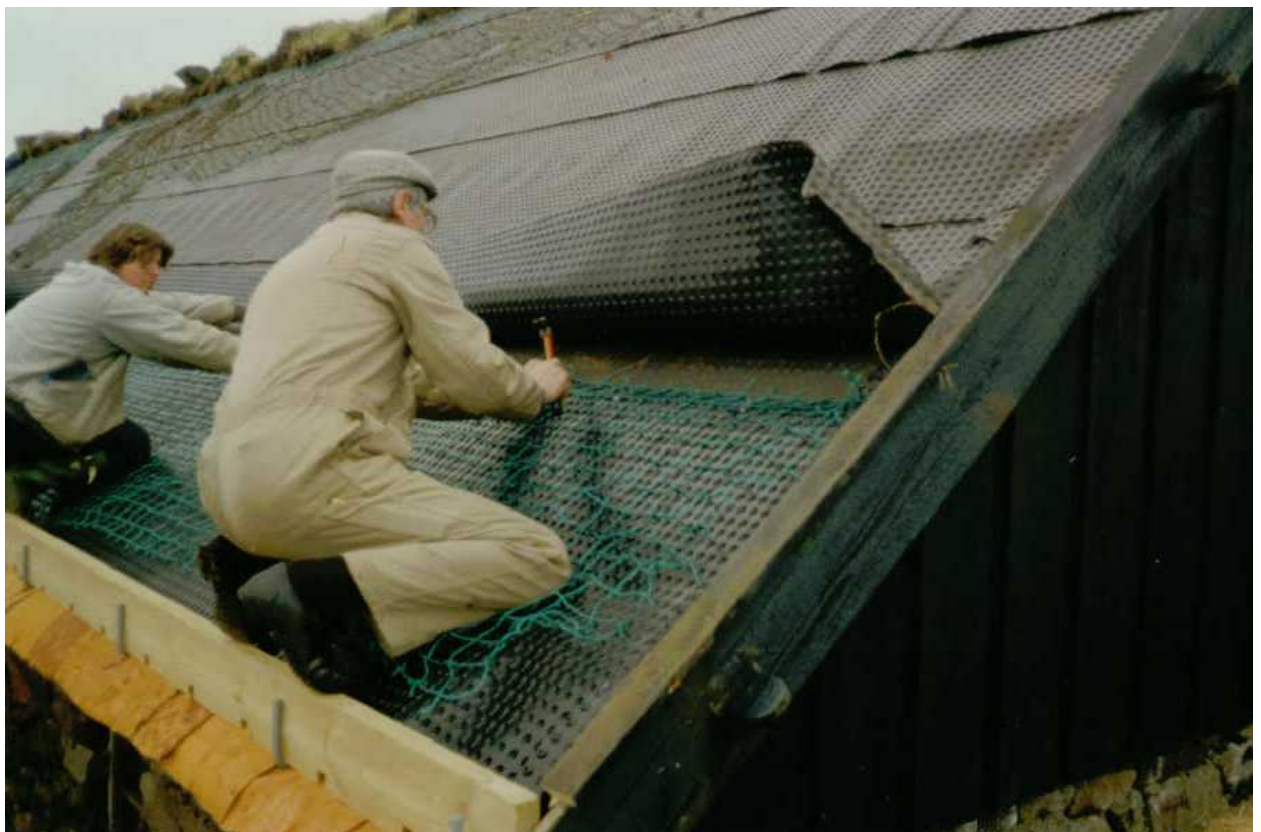
Fig. 7. The turf retainer board in place.
