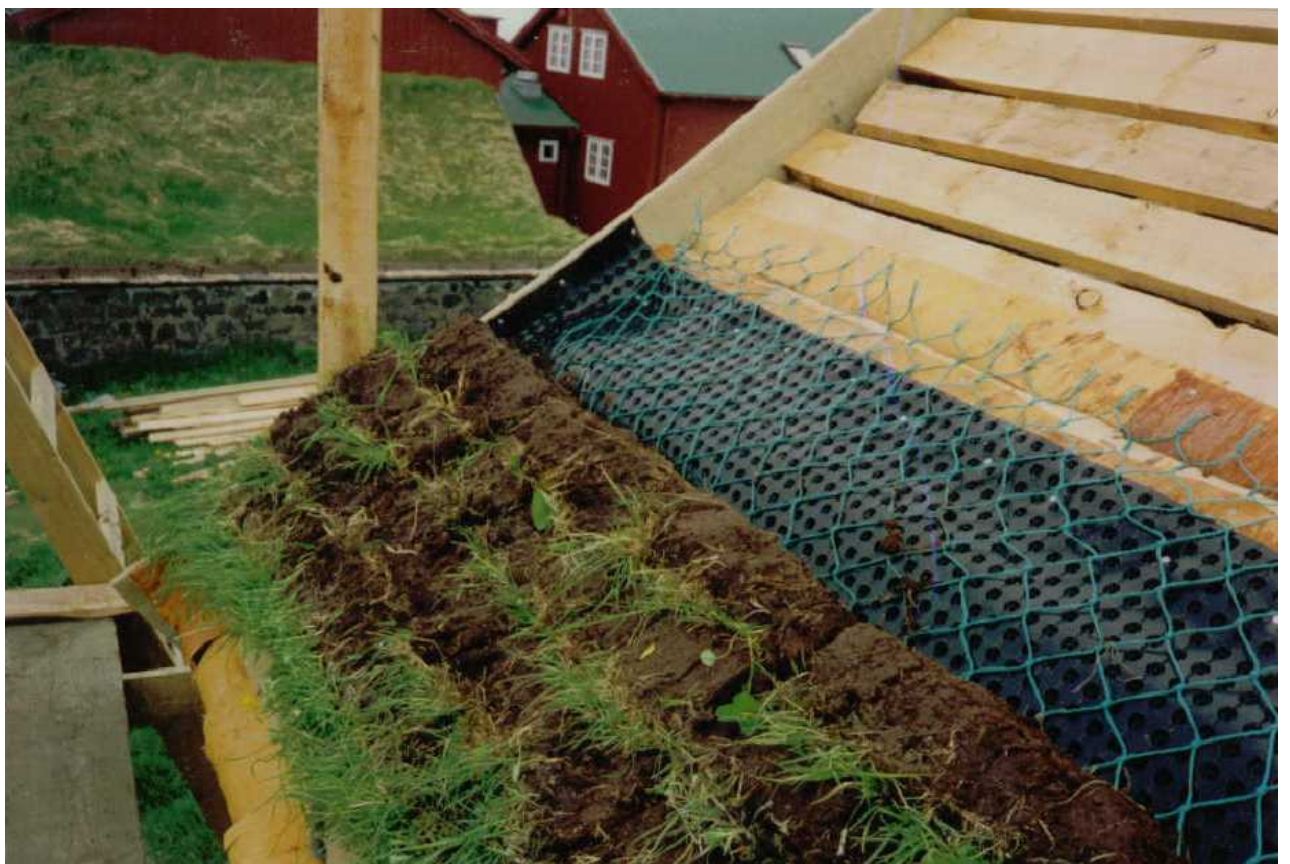
Fig. 19. The roof, birch bark, knobbed plastic sheeting, trawl-netting and lastly the turf.
