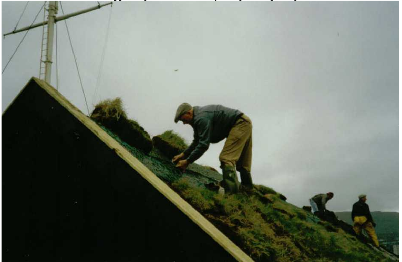
Fig. 9. Trawl netting is laid lengthwise along the ridge and securely tied to each side-netting section.
