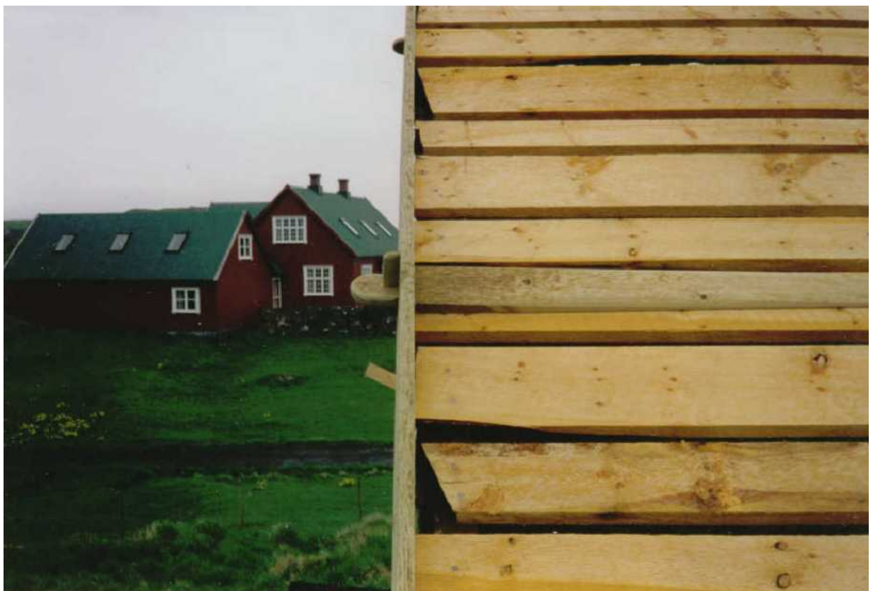
Fig. 17. The locking pins for holding the gable bargeboards can be an integrated part of the roof construction as depicted, or separately festooned on to the roof laths.
