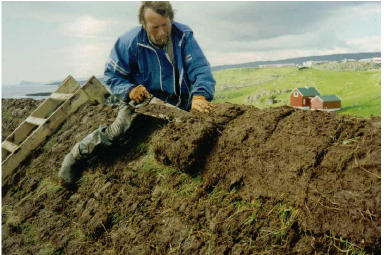
Fig. 18. A double layer of sods are laid upon the roof ridge.
