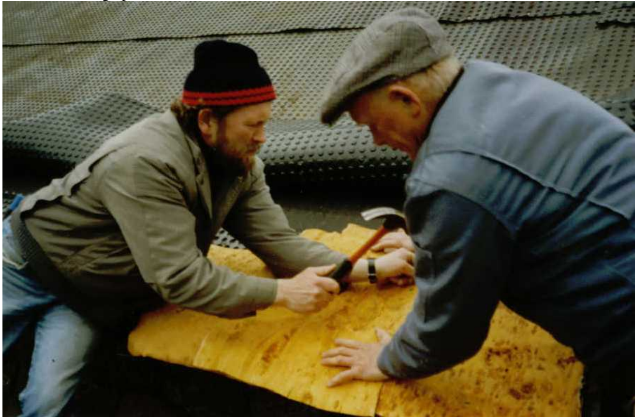
Fig. 5. Bark being fastened with roofing nails on its upper edge.
