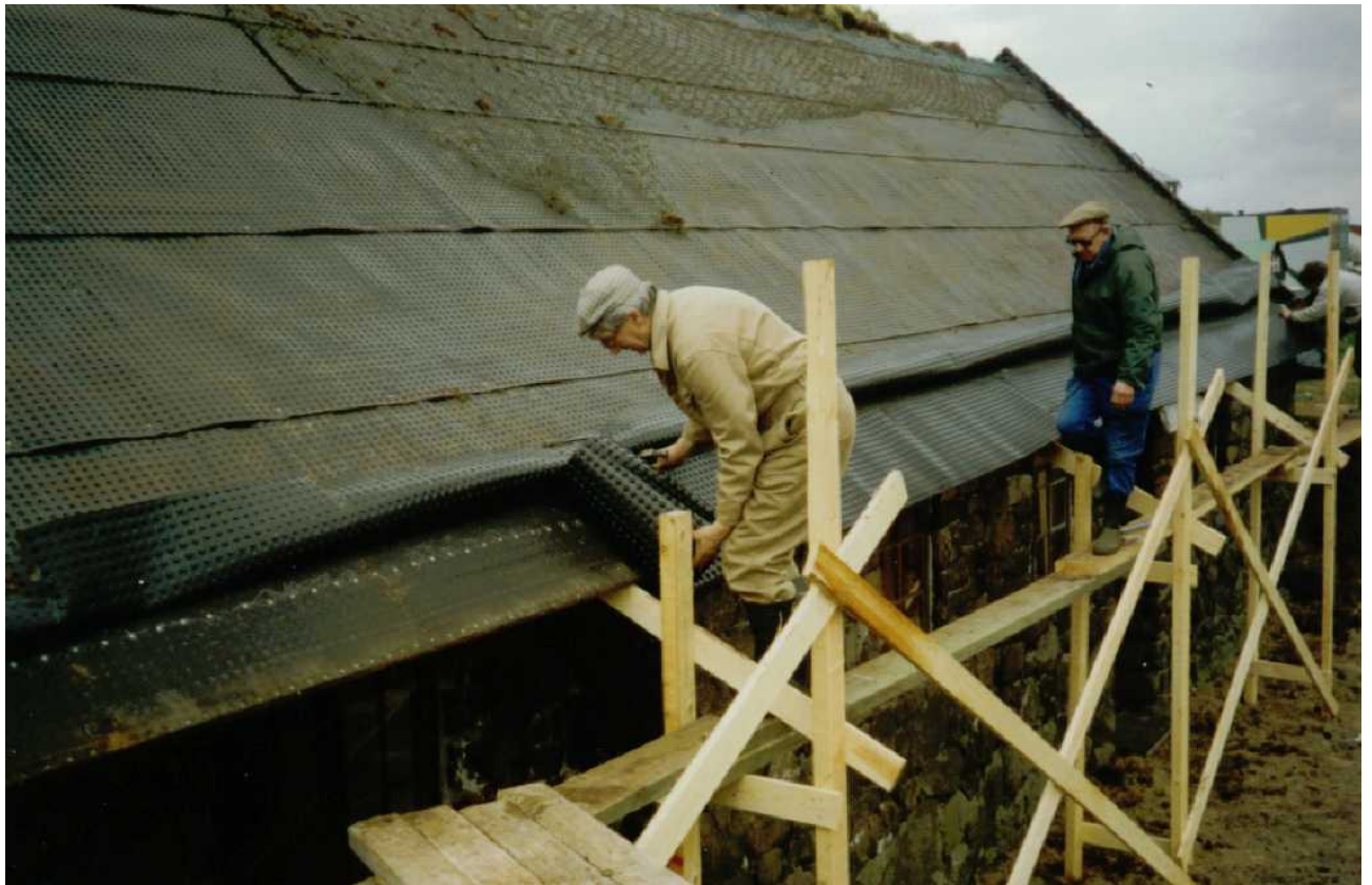
Fig. 1. Knobbed plastic sheeting being laid.
