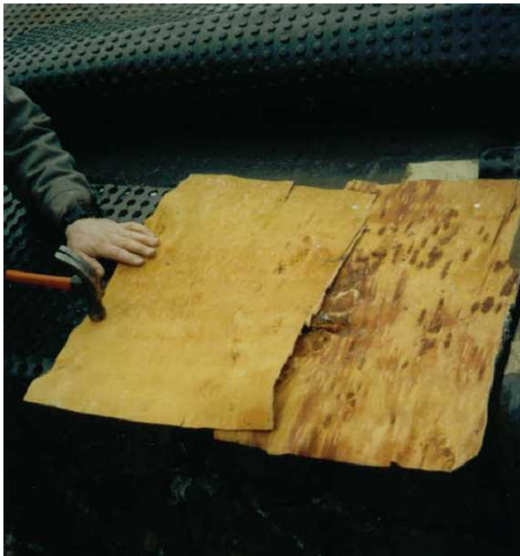
Fig. 3 Birch bark bent upward and festooned to the gable bargeboard.
