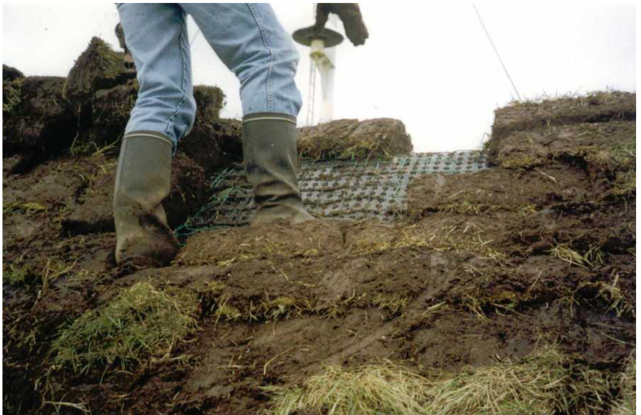
Fig. 13. The sods are app. 15 cm high, or app. the depth of a spade blade.
