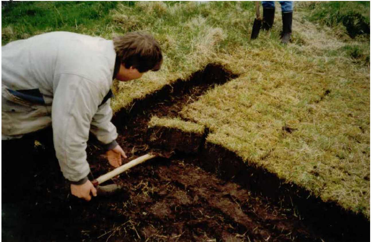
Fig. 13. The sods are app. 15 cm high, or app. the depth of a spade blade.
