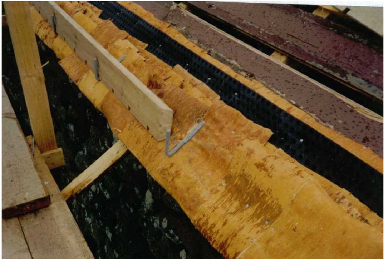
Fig. 16. It is most aesthetically pleasing to the eye, if the distance between the frost holes correspond to the turf retainer irons.
